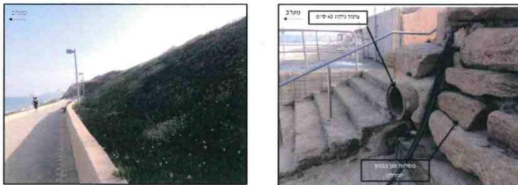
Figure 18 : regulated slope stabilized by plantation above the promenade and rain runoff outlet of Ha'Tzuk Beach
